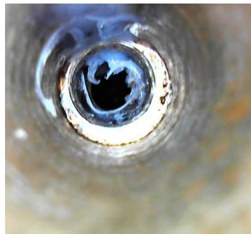
水路清洗后 Cooling channel after cleaning
